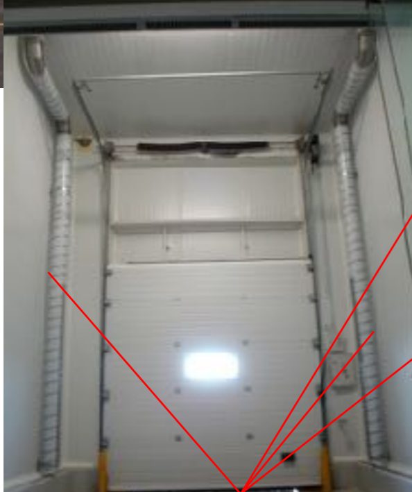
Position process air inlet close to the truck door.
